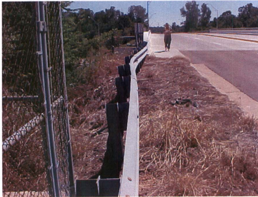
APPROACH #2, RIGHT GUARDRAIL HAS COLLISION DAMAGE
