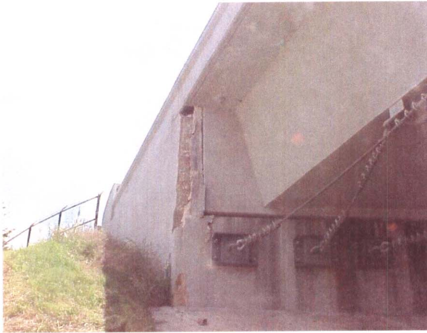
ABUTMENT #1, RIGHT SIDE OF BACKWALL SPALLED TO STEEL
