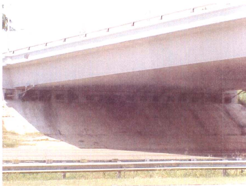
ABUTMENT #1, LEFT SIDE OF BACKWALL SPALLED TO STEEL
