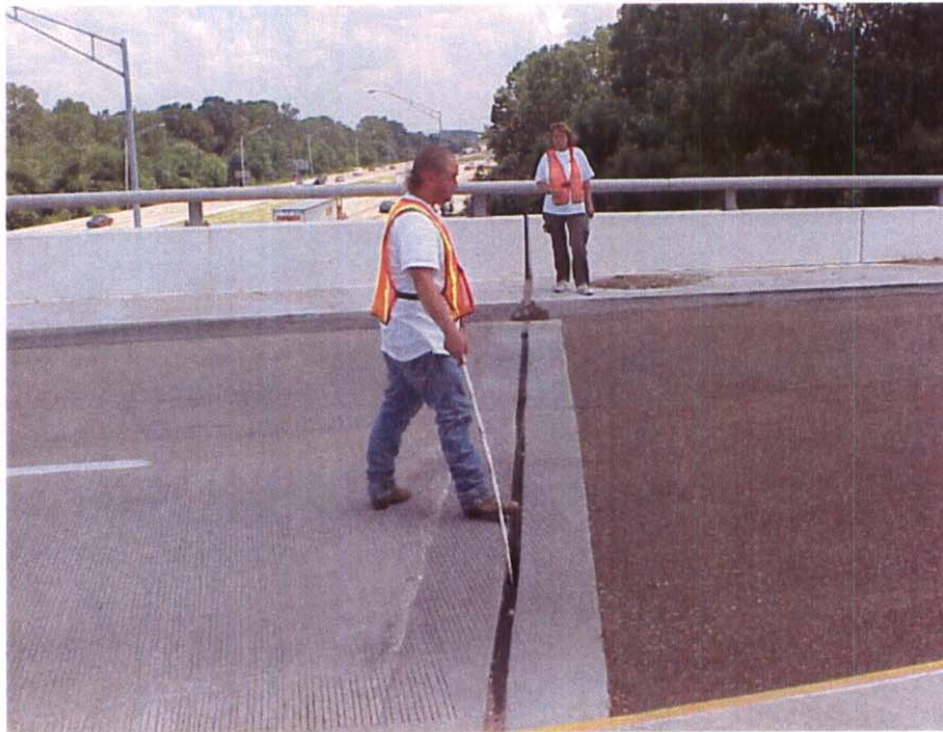
APPROACH #1 WITH JOINT MATERIAL MISSING, TYPICAL OF APPROACH #2
